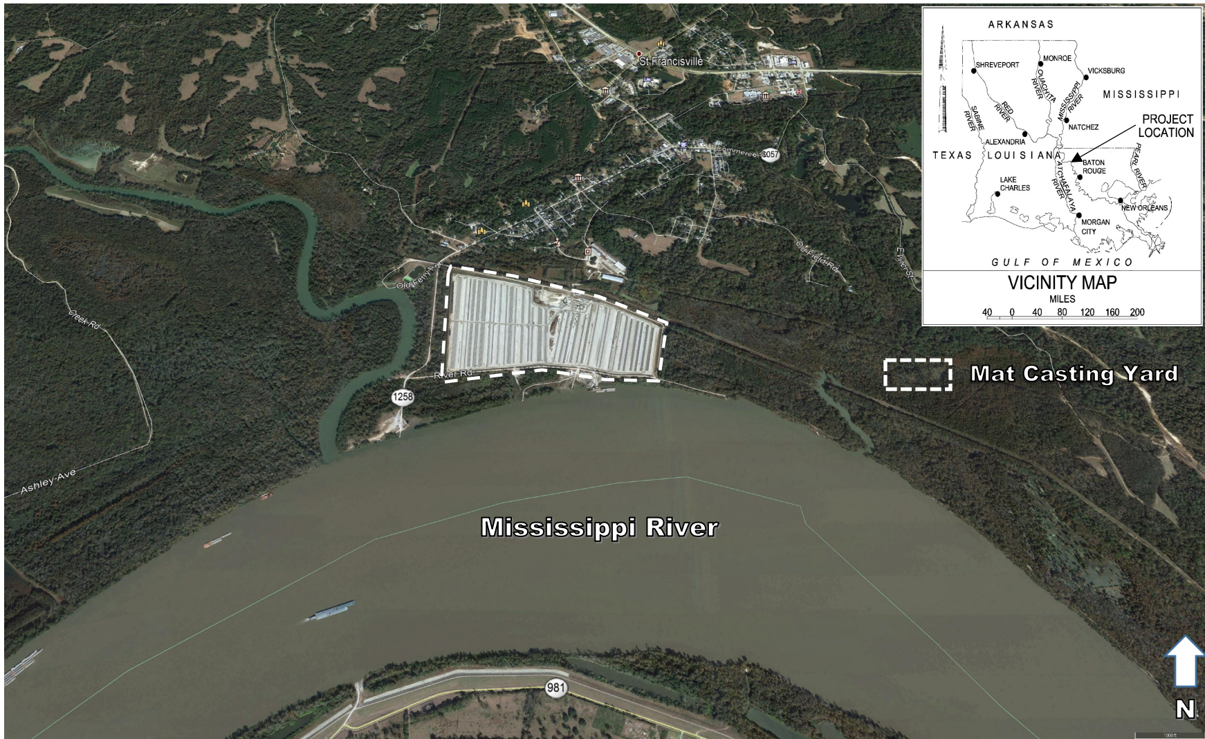
Figure 1: St. Francisville Mat Casting Yard, West Feliciana Parish, Louisiana
