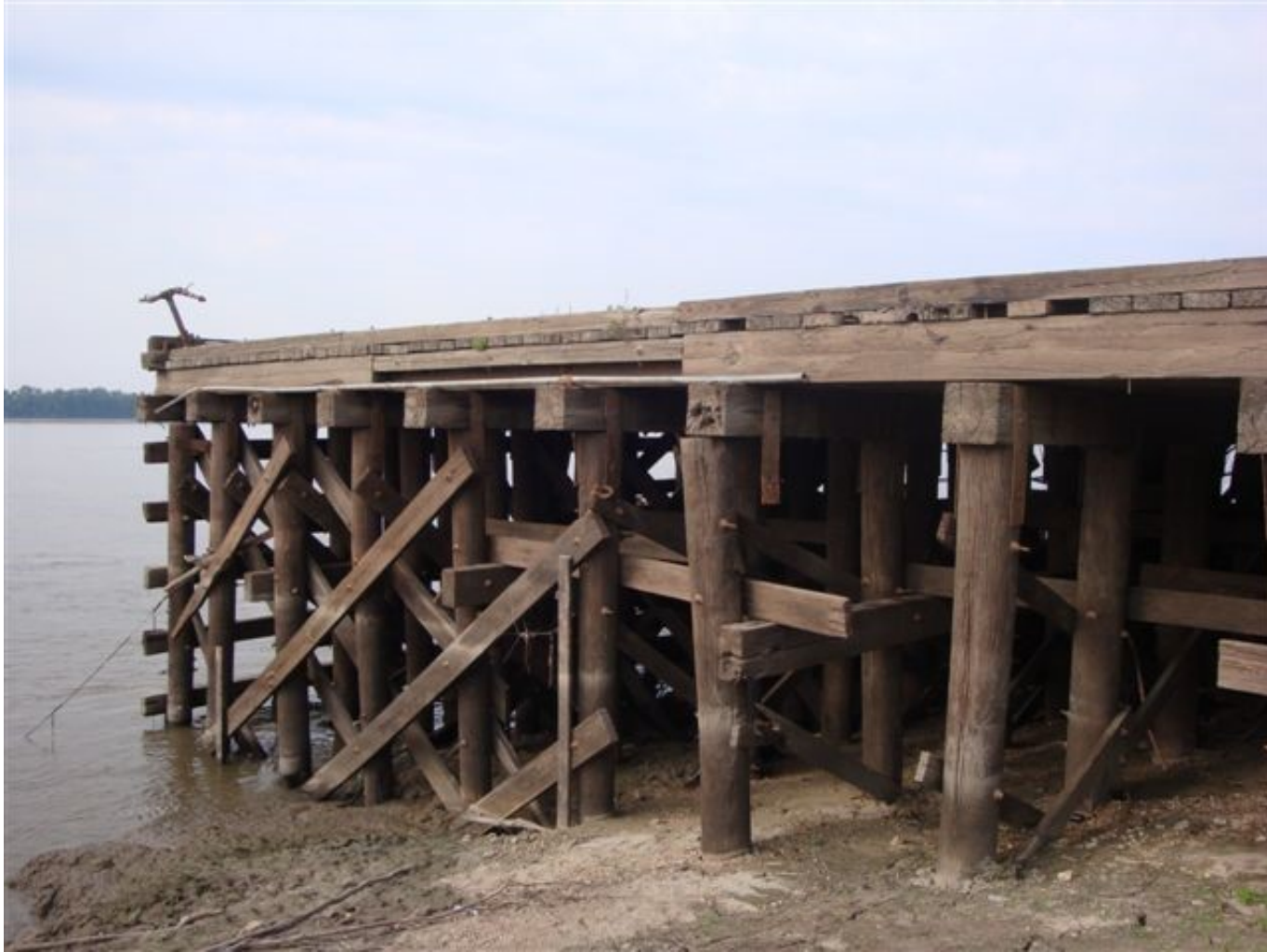
Figure 3: St. Francisville Mat Casting Yard, Old Load-out Dock (To Be Demolished).
